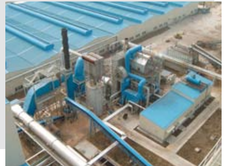
Plant area, Lishui
