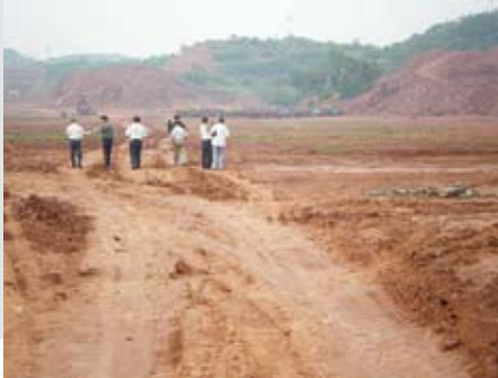
Site levelling works mid 2008
