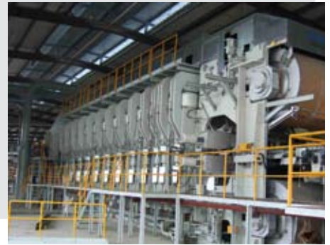
CPS during installation
