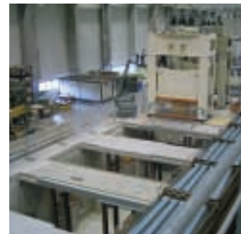
Installation of the press line at Polynorm Grau
