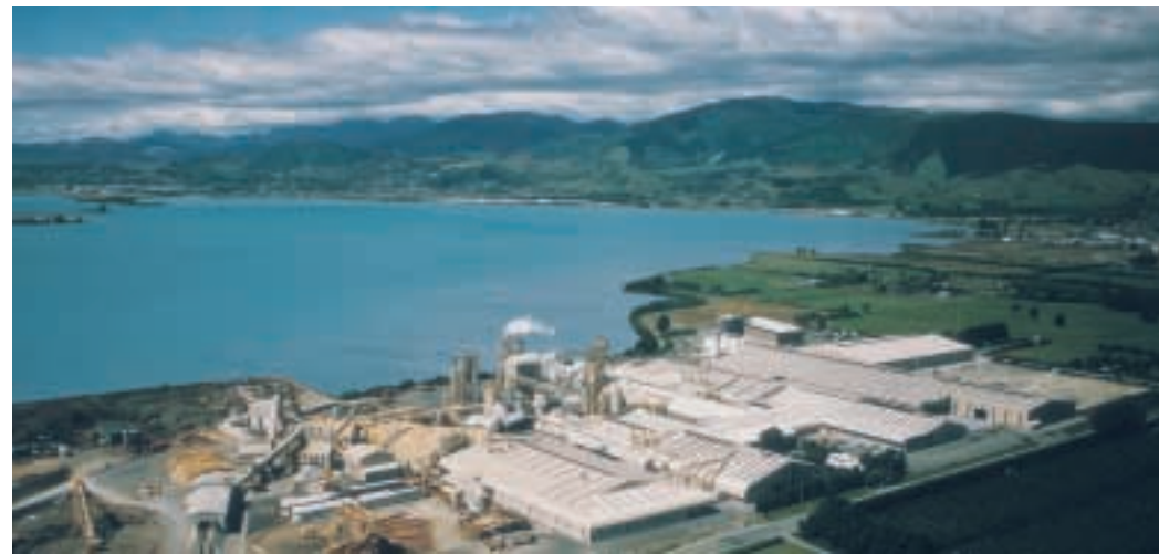
Continuous LVL production plant of Nelson Pine
